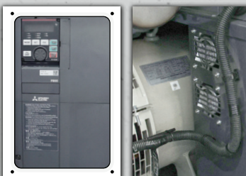
7 | 480V Variable Frequency Drive with Cooling Fans
