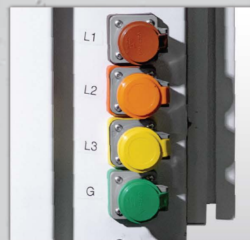
2 | Convenient CAM-Lok Input Connection 3Φ 480V Cam-Loks™
