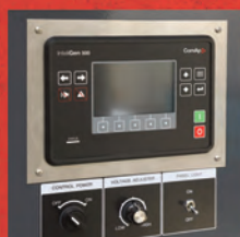
Parallelling Control Panel
