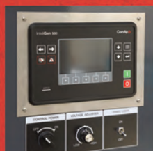
Parallelling Control Panel
