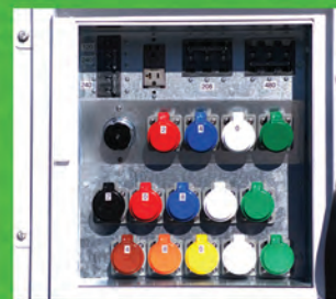
Single-Phase (110/240V) and Three-Phase (208/240/480V) Receptacle Outlets
