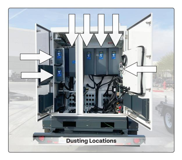
Compressed air should be used to remove dust and debris from the EBOSS<sup>™</sup>. Do not make contact between the air nozzle and the sensitive electronics of the EBOSS<sup>™</sup>, as damage can result.
